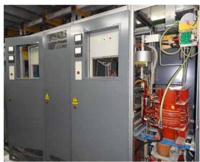
Fig. (5.3)10. Reversible current power supplies IST for IC channels.
