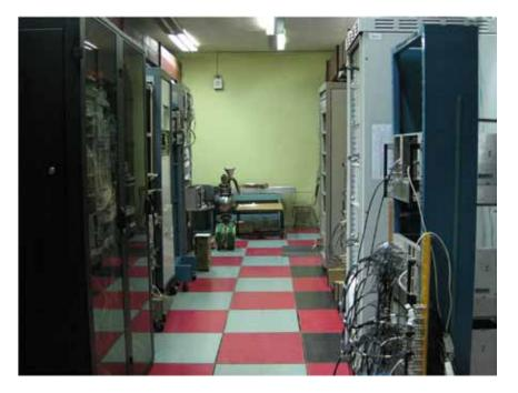
Fig. (5.3)3. Master oscillator-power amplifier at radio equipment room of IC.
