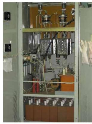
Fig.(5.11)3. Anode modulator.
