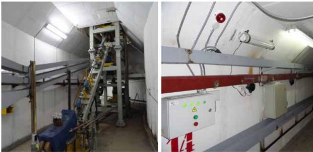
Fig. (5.3)6. Elements of downtake channel to VEPP – 3 with coolant circuit.
