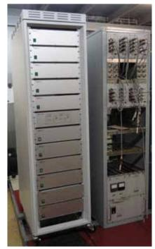
Fig. (5.3)9. New rack of ion pumps power supplies.
