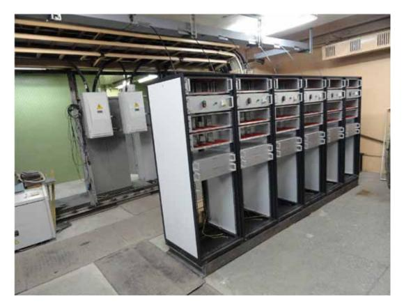
Fig. (5.3)11. New racks of pulse power supplies for the IC channels.
