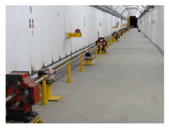
Fig. (5.3)5. General view of channel to VEPP – 2000 with magnetic elements, cable trays and ground loop.
